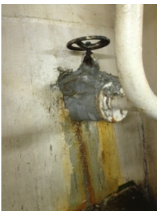
Picture 7 – Leaking Overboard Repaired With Cement
