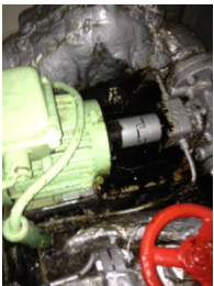
Picture 6 – Leaking Fuel Pump
