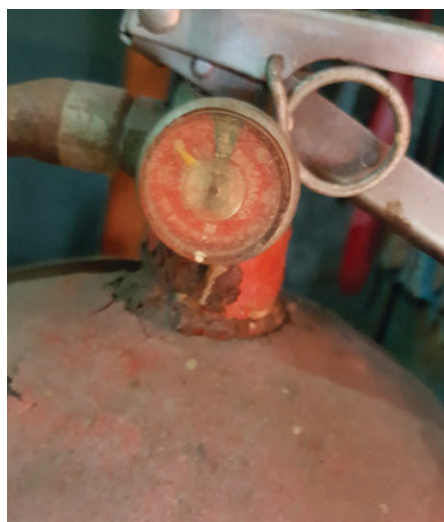
corroded fire extinguisher with leak and gauge showing empty
