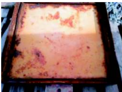
Hatch Cover with Missing Gasket
