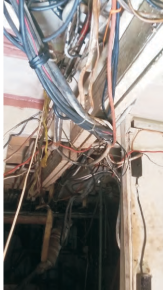
Lose electrical cables in machinery space
