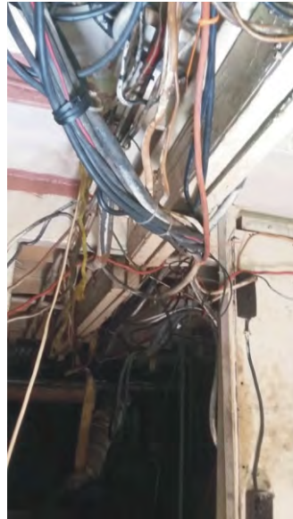
Loose electrical cables in machinery space
