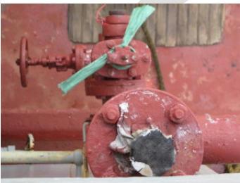
Pictures 4 – Fire Hydrant seized and hand-wheel missing
