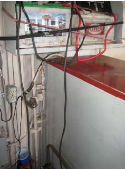
Picture 2 – Emergency lighting batteries discharged
